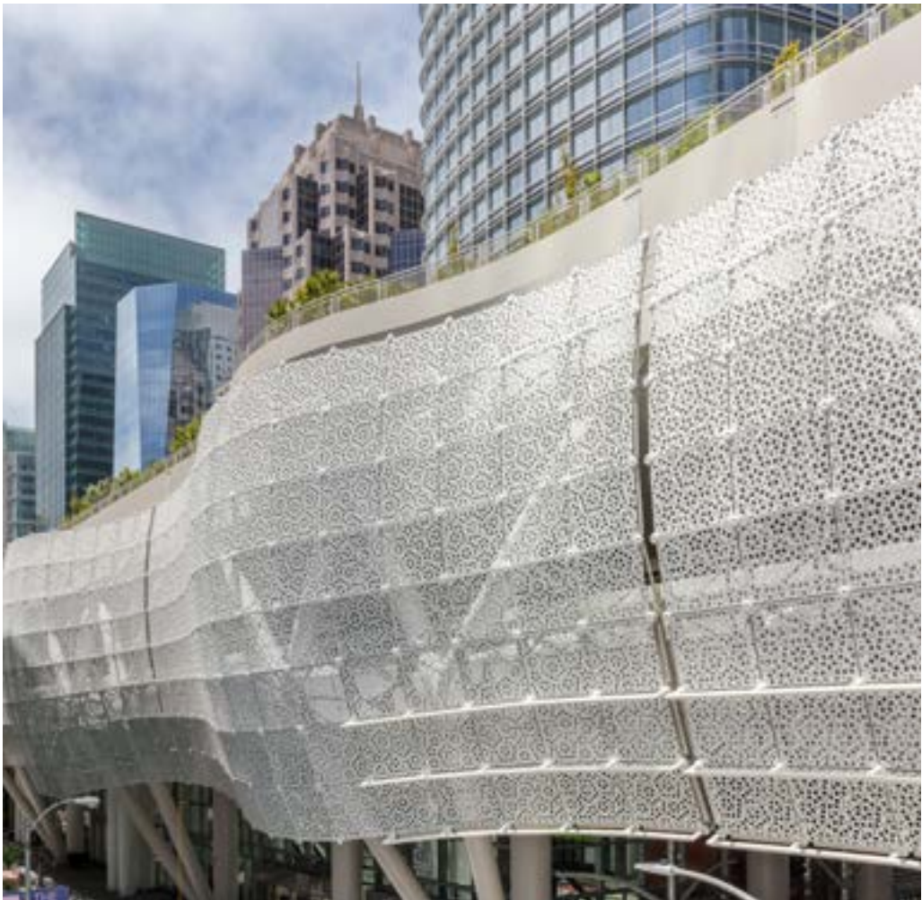
Salesforce Transit Center is wrapped with a white aluminum screen, perforated with an intricate pattern devised by mathematician Roger Penrose that protect birds from impact and allow views out for users of the building.
