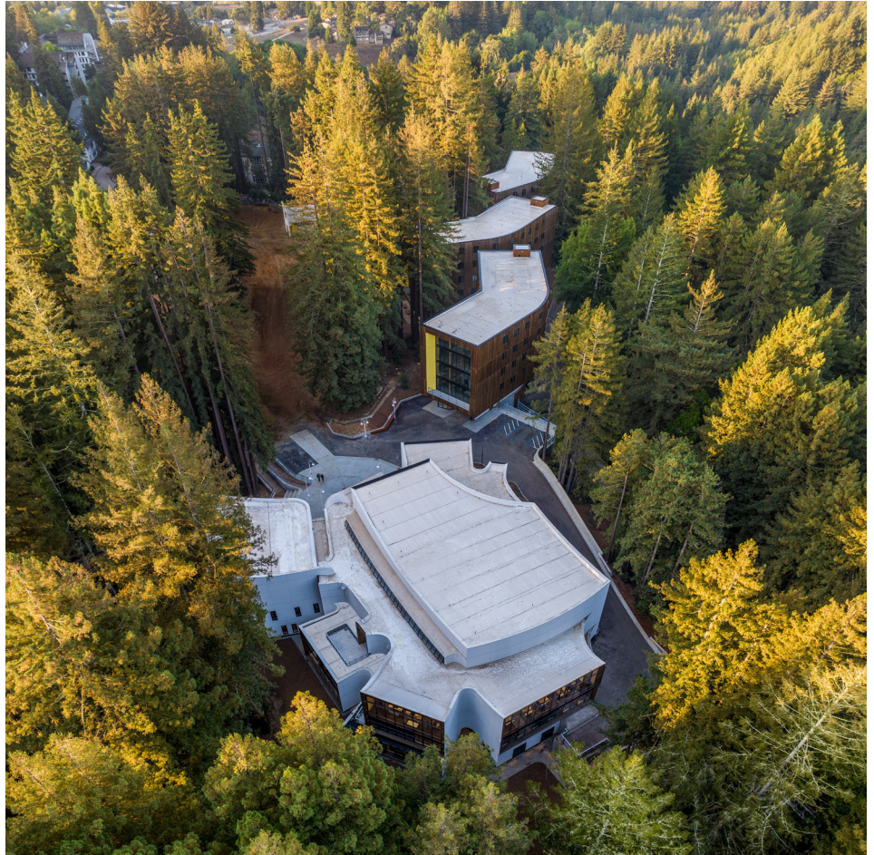
Atelier Ten coordinates with every project team to develop a project-specific timber procurement strategy. FSC certification was prioritized for mass timber elements and exterior cladding at Kresge College, UC Santa Cruz. With Studio Gang Architects
