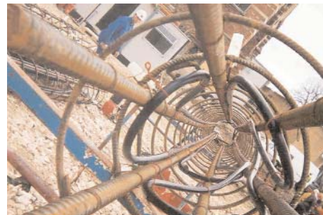
Water pipes run through the piling reinforcement cages, turning the concrete foundation elements into heat exchangers for the building (above); Conditioning strategy (below)
