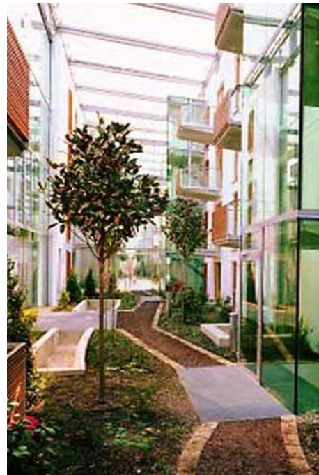
A moveable membrane within the inflated roof shifts position to control solar gain within the microclimate zone (above); The Microclimate Zone nestles between the housing blocks, while sliding solar shades screen the exterior facades (below)
