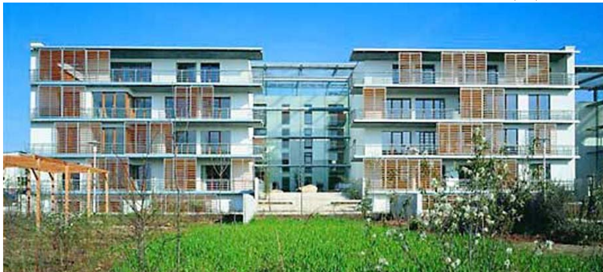
A moveable membrane within the inflated roof shifts position to control solar gain within the microclimate zone (above); The Microclimate Zone nestles between the housing blocks, while sliding solar shades screen the exterior facades (below)
