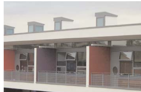
Classrooms with wind chimneys (above)
