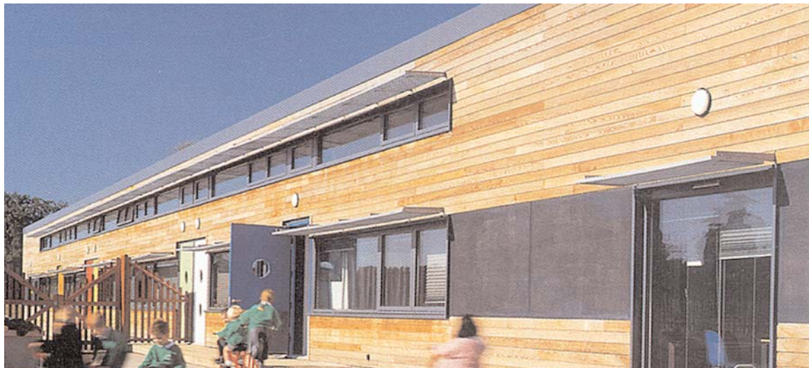
External panels use a timber breathing wall construction. Glazing is optimised for daylight (below)
