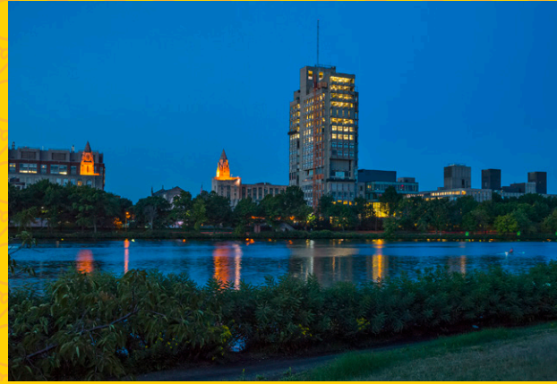
▲ School of Law Renovation and Addition, Boston University
