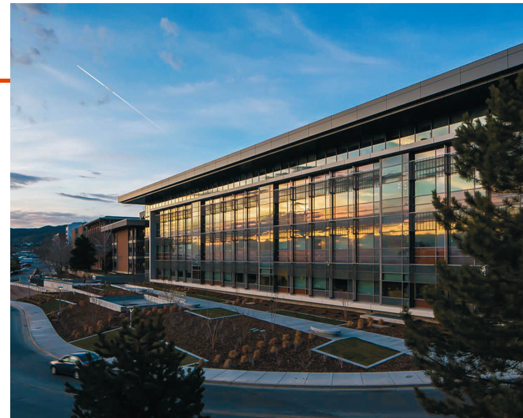
The final façade of L.S. Skaggs Pharmacy Research Institute, reflecting the local landscape
