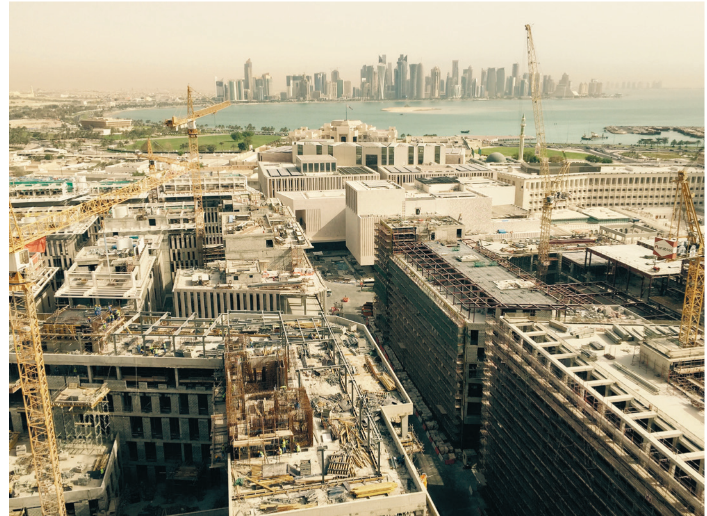
Construction of Downtown Doha well underway, as of April 2015
